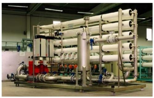
The Lofsdalen nanofiltration plant consists of 10 pressure vessels, each containing four FILMTECTM elements. The vertical metal cylinder is the housing for the cartridge filters. The two vertical boxes at the left are the frequency controllers for the recirculation pumps below. All pipework is stainless steel. (Photo courtesy of HOH Water Technology.)
